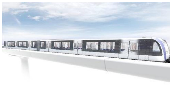
TOULOUSE, FRANCE – Metro system – €470m
